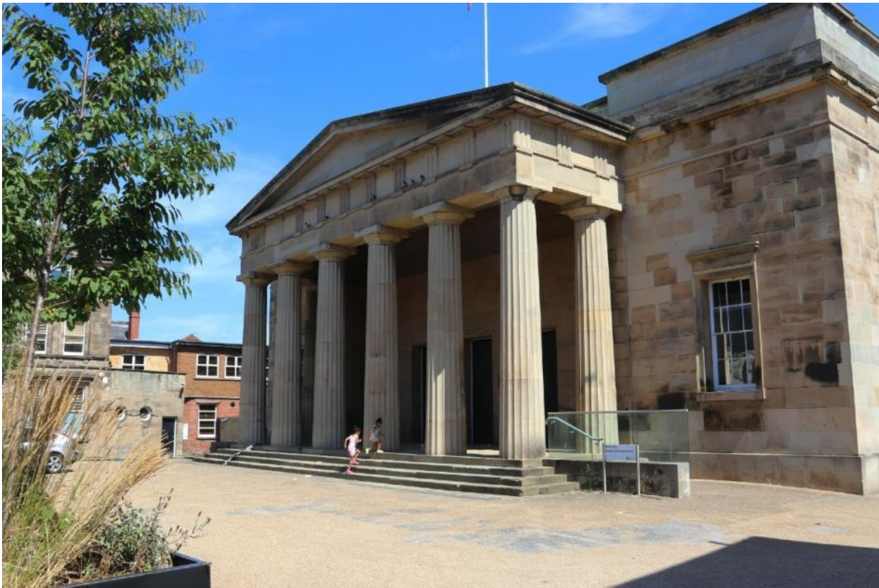
Fig 11: Front of Shirehall building
